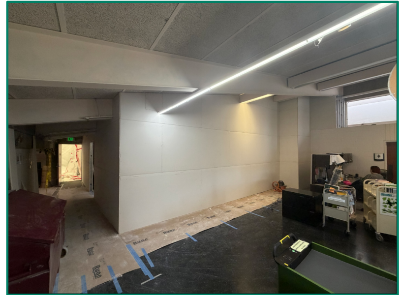
Farmington Hills: Temporary wall enclosure installation on-going
