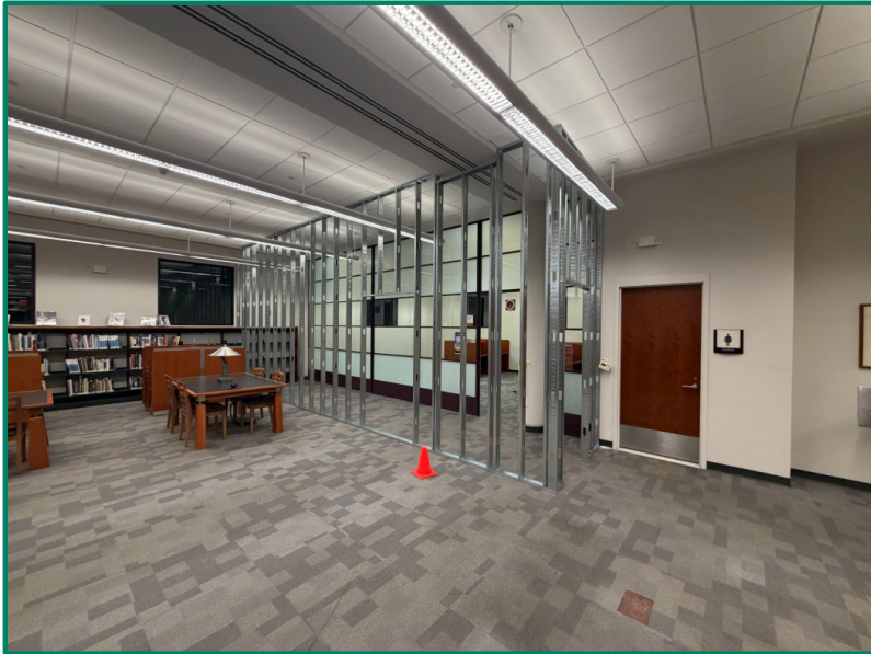
Farmington Hills: Temporary wall enclosure installation on-going
